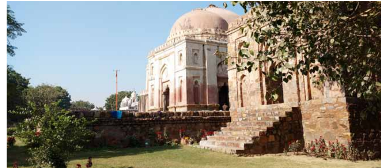
The isolated tomb is accessed by lower plinth but by climbing 9 steps. Its plinth level matches that of the upper plinth
