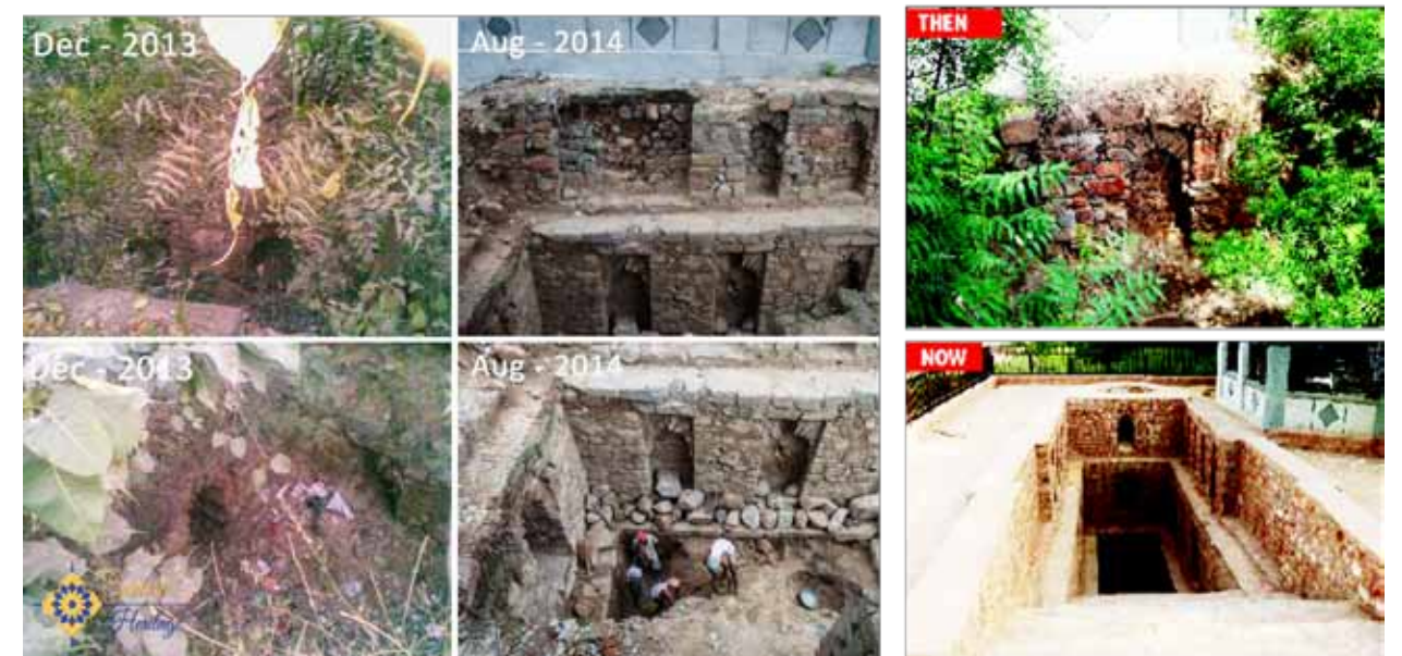
Pictures of the baoli before & after restoration
