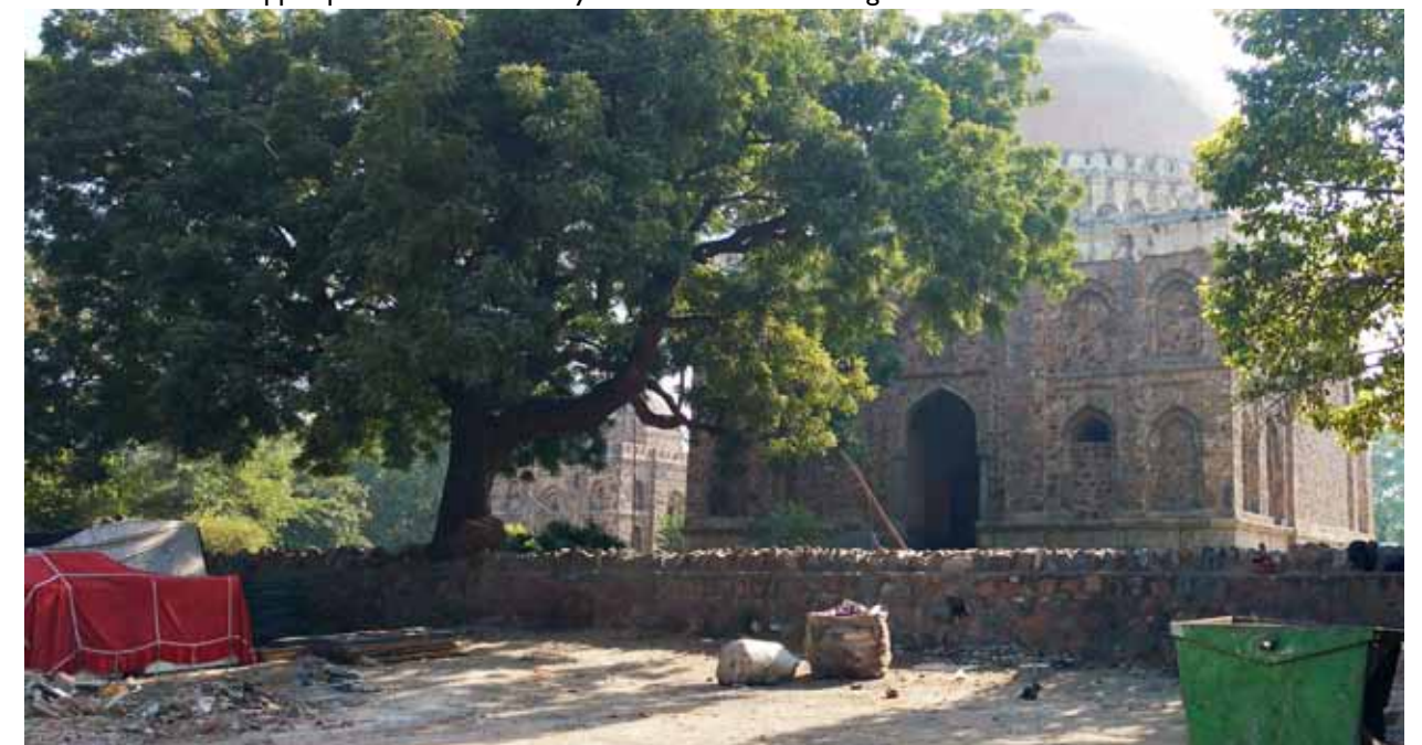
Rear view of the upper plinth's stone rubble retaining wall.
