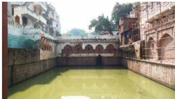
The structures surrounding the baoli are in a state of distress though revival of the old structures and removal of encroachments is still in process
