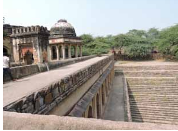
It has a series of steps forming four stages, each in descending size, with floors at each stage, leading to the water level from the surrounding ground level
