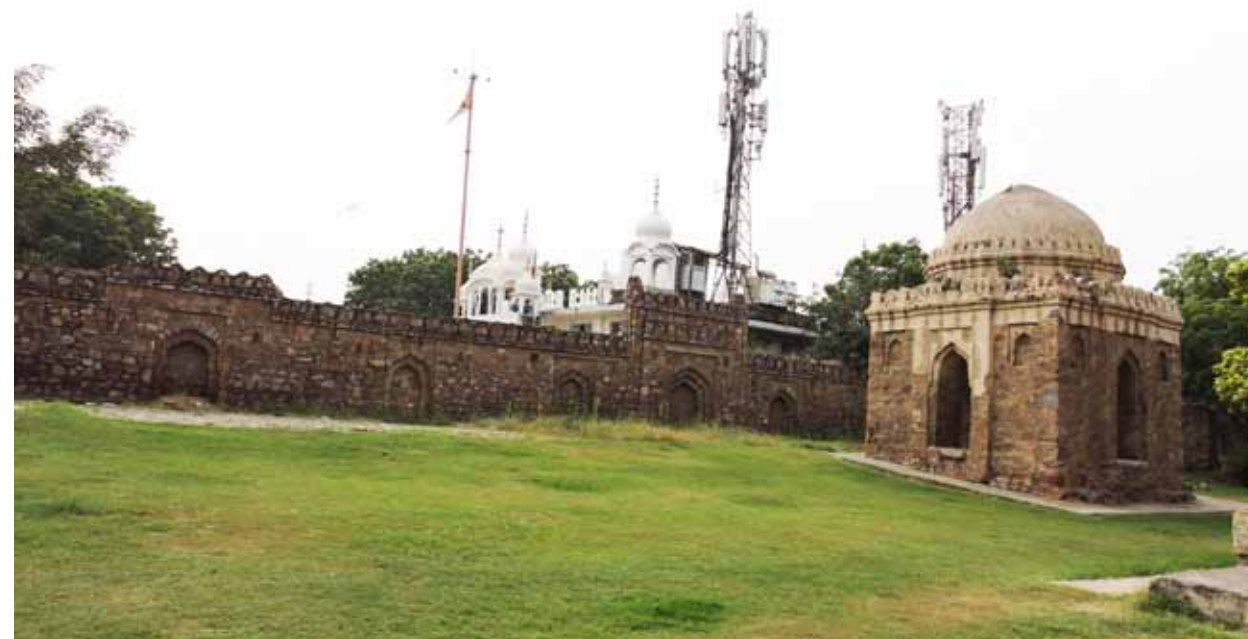
Localised slopes created on the site to drain surface water
