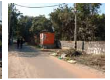
Transformers at the edge of the monument complex
