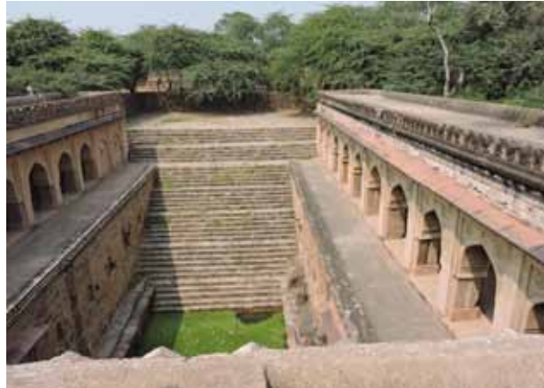
It has a series of steps forming four stages, each in descending size, with floors at each stage, leading to the water level from the surrounding ground level
