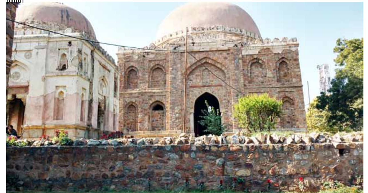
The tombs on the upper plinth are enclosed by a stone rubble retaining wall.
