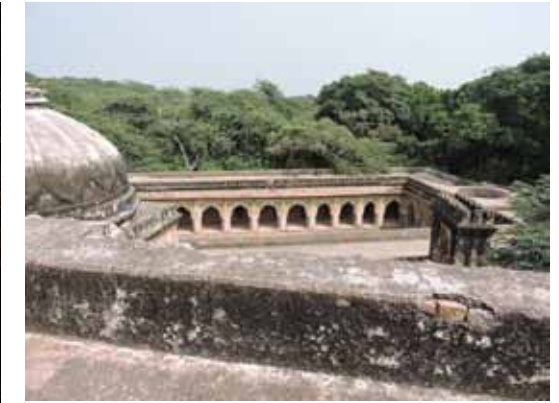
There are rooms at each floor which once provided a cool resting place for people
